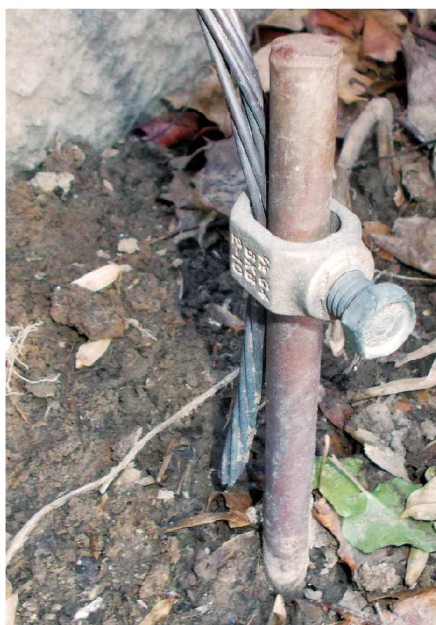
Figure 5 — A ground rod and acorn clamp securing stranded #6 AWG ground wire. This is typical of clamped connections that are replaced and upgraded by the welded Uni-Shot connections.
