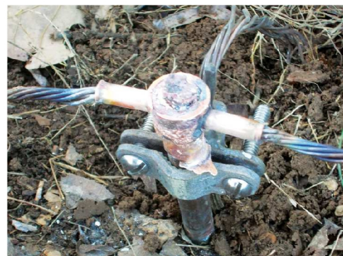
Figure 7 — The final welded connection. An additional ground conductor is clamped to the rod. This connection will not be buried.
