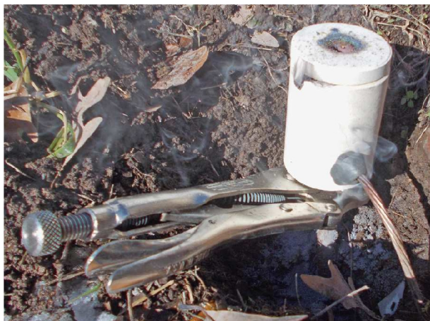
Figure 6 — The Uni-Shot in action with mold sealer around the ground rod and both wire sleeves. Clamping pliers support the crucible so it is vertical.
